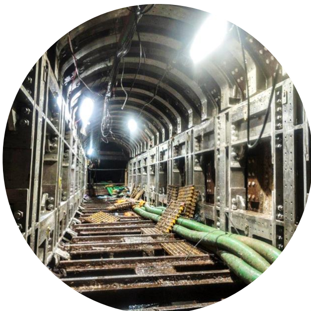
Support structure being installed in the sewer.
